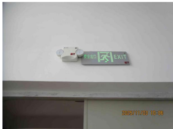
Safety exit sign and emergency light.jpg
