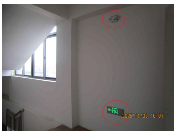
Evacuation staircase with emergency lighting and evacuation sign.jpg
